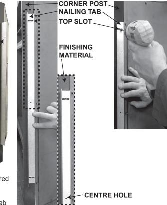
**5.4.4** To determine the final location of the nailing tab you must first determine the thickness of your fin-
